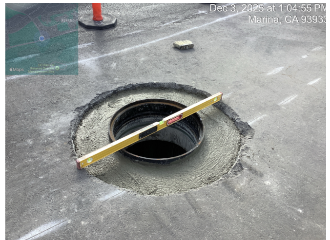
Checking for proper height and placed concrete collar around manhole cone
