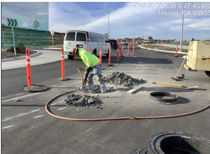
Removing asphalt around manhole to raise up to final grade (aka "raising iron")
