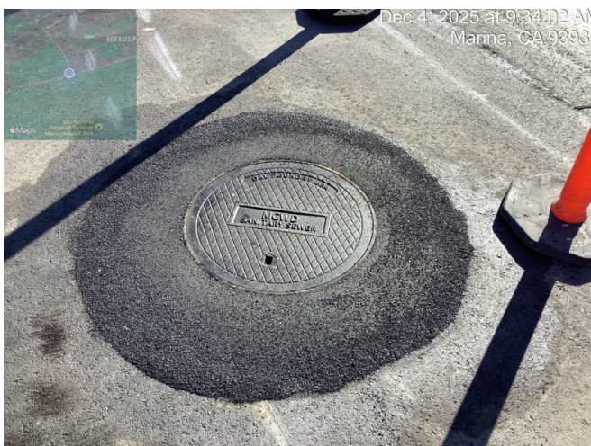
After concrete has cured, replace asphalt around manhole cone to grade
