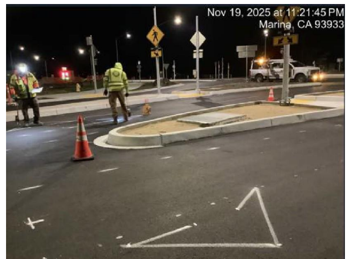
Crew performing layout for pavement markings at Abrams Drive roundabout
