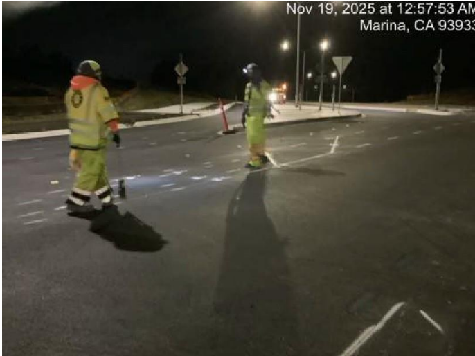
Crew performing layout for pavement markings at Abrams Drive roundabout
