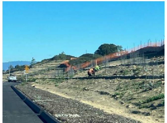
Crew planting trees on slope between Imjin Road and Marina Heights Drive
