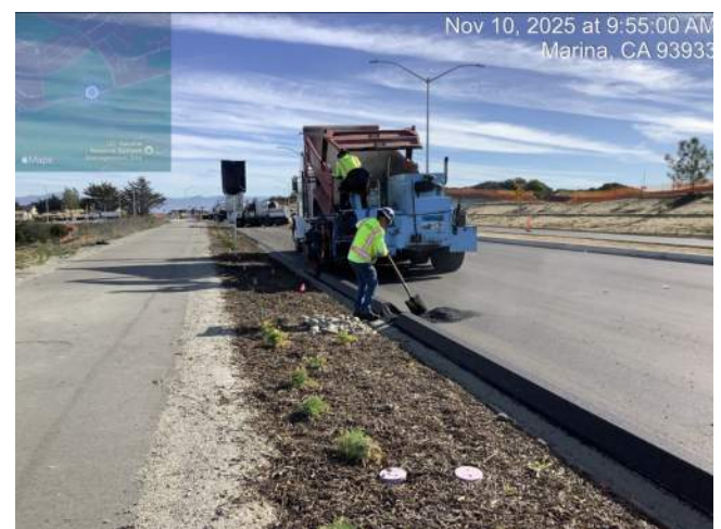
Curb machine installing asphalt berm
