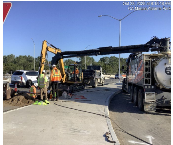
Working on water main repair
