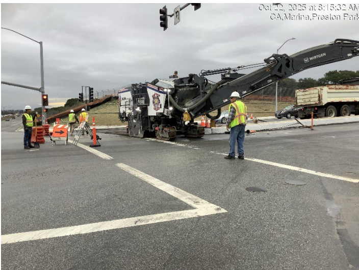
Grinding asphalt to prepare roadway for upcoming paving
