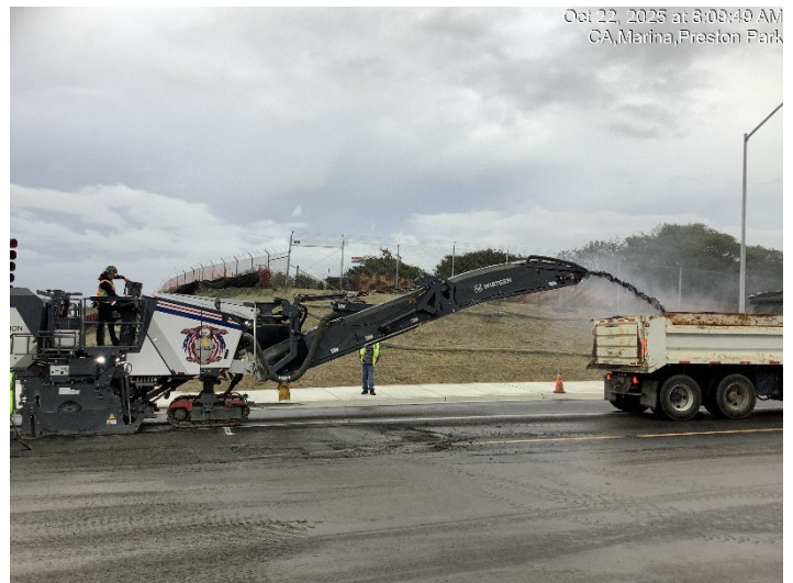
Grinding asphalt to prepare roadway for upcoming paving
