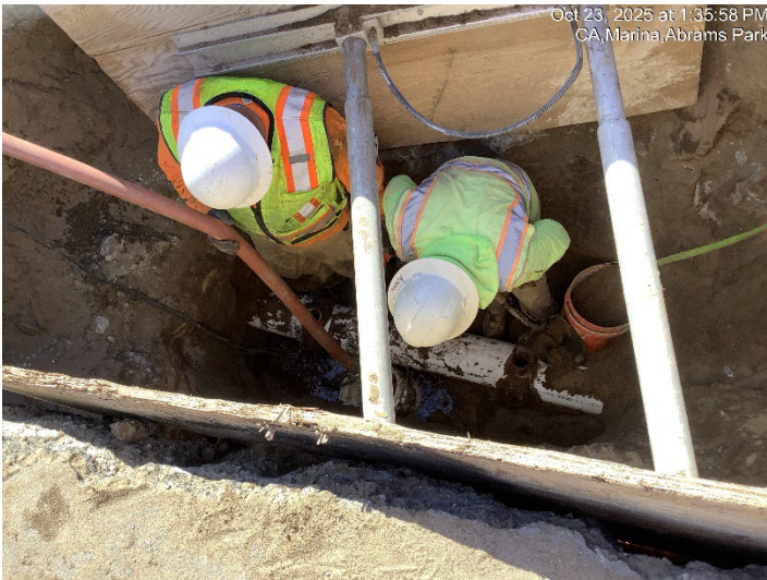
Water main repair
