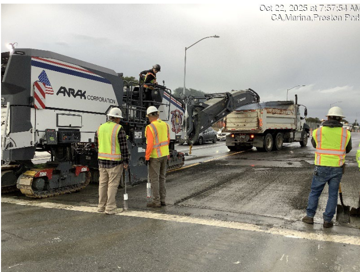
Preparing roadway for upcoming paving
