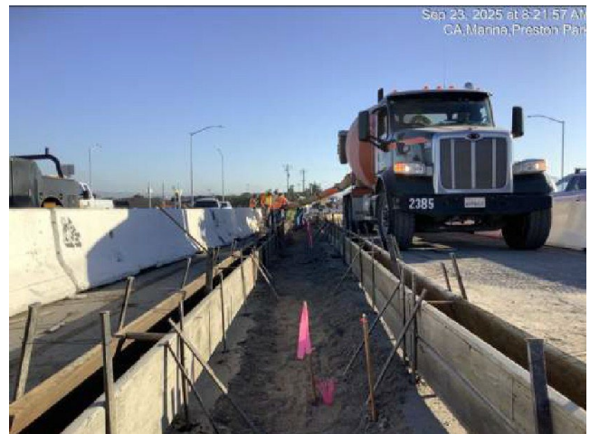
Forming and placing concrete for median curb west of Preston Drive
