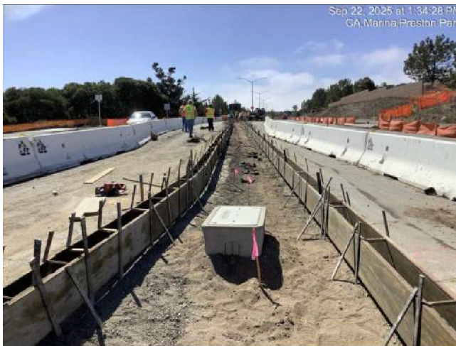
Forming and placing concrete for median curb west of Preston Drive
