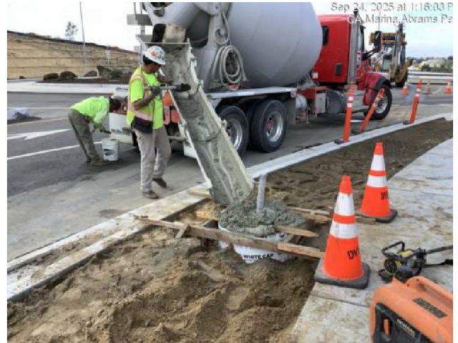
Forming and placing concrete for streetlight foundation west of Preston Drive
