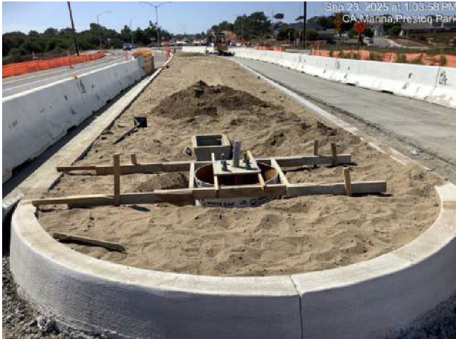
Forming and placing concrete for streetlight foundation west of Preston Drive
