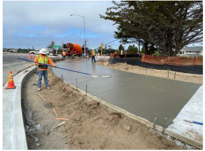
Placing concrete for sidewalk at Marina Heights Drive
