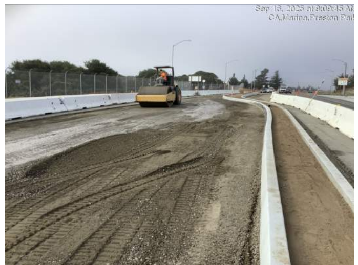
Prepping in-fill area for pavement between Army Reserve and Reservation Road
