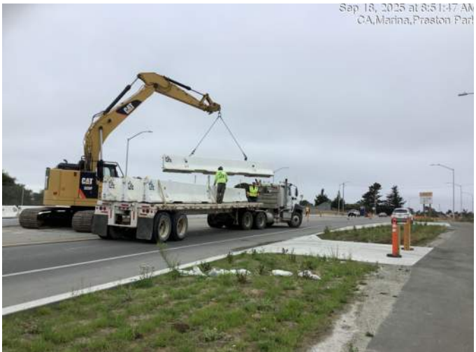
Removing concrete barriers near Preston Drive
