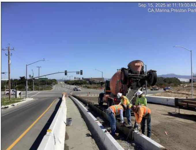
Placing concrete for median curb between Army Reserve and Reservation Road
