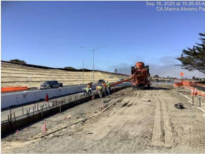
Placing concrete for curb & gutter at Marina Heights Drive
