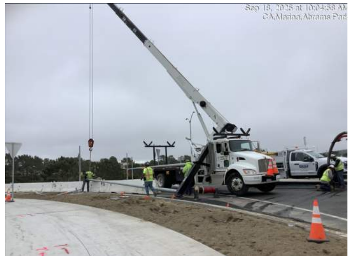
Wiring/installing streetlight at Abrams Drive (north)
