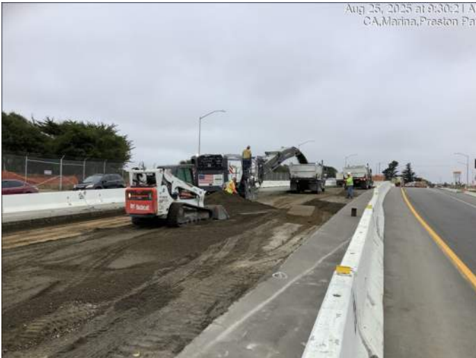
Grinding and removing temporary pavement near Reservation Road (left) and Abrams Drive (right)
