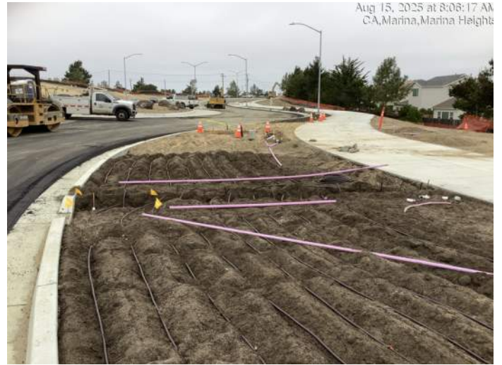
Installing elements of the irrigation system for plant establishment
