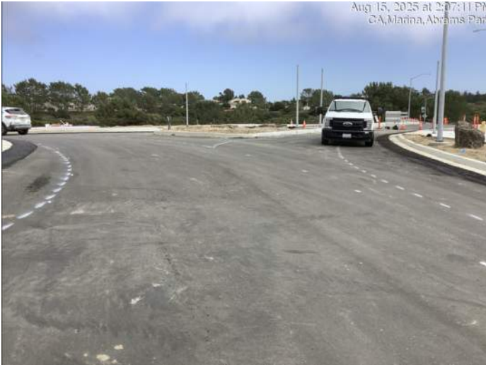
Beginning of striping layout (aka "cat tracking")
