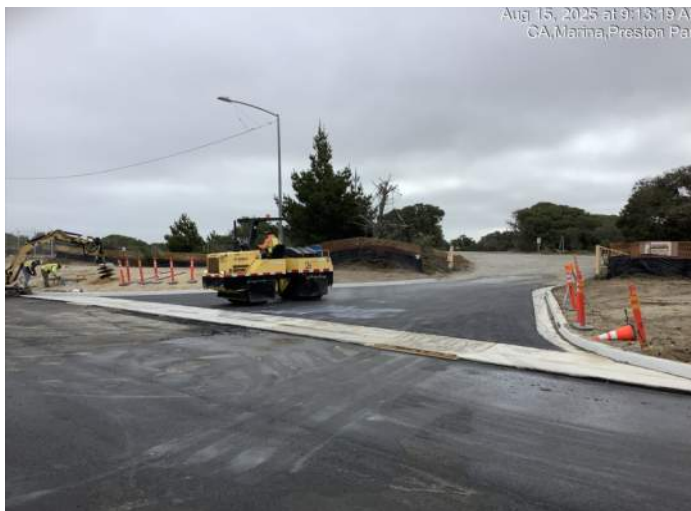
Asphalt paving for Chapin yard driveway
