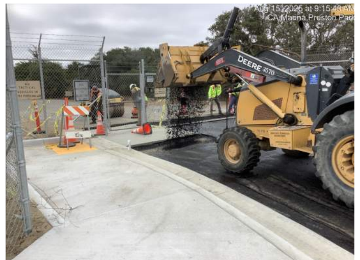
Asphalt paving Army Reserve driveway
