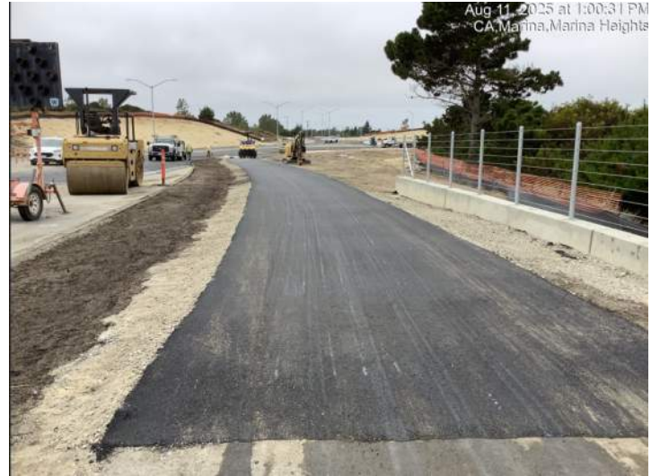
Asphalt paving for bike/ped path near Imjin Road
