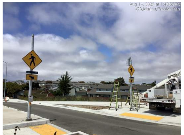
Connecting electrical and installing Rapid Flashing Beacons (RFB's) at pedestrian crossings
