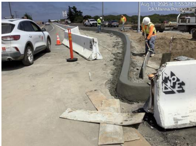
Placing concrete for median curb
