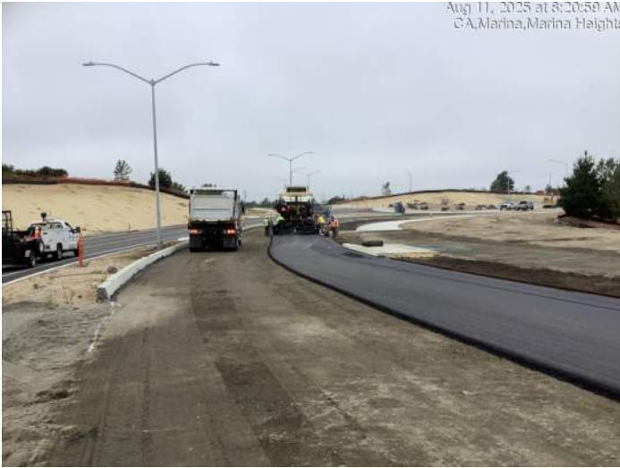
First layer of asphalt paving near Imjin Road
