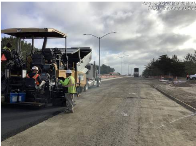
Paving first layer of asphalt starting at Abrams Drive (south) heading to Reservation Road
