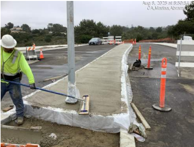
Concrete placement for median in-fill at Abrams Drive
