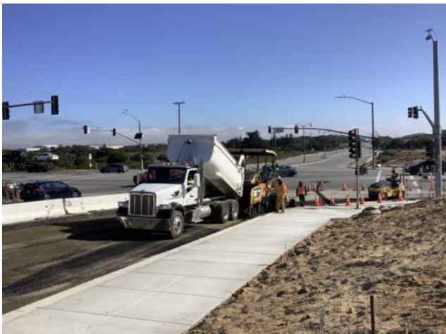
Tying into existing roadway at Reservation Road
