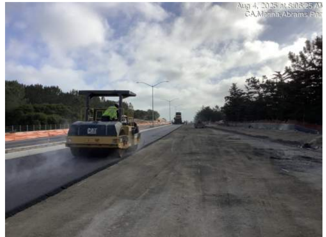
Paving first layer of asphalt starting at Abrams Drive (south) heading to Reservation Road
