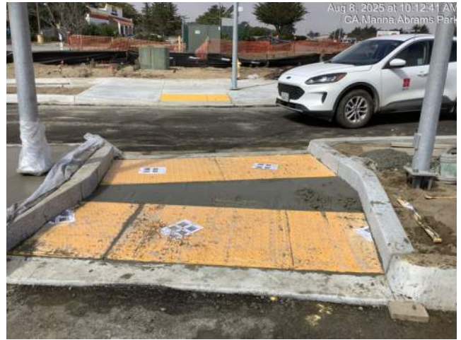
Concrete and "tactile domes" (yellow bumpy plates) for pedestrian crossing at Abrams Drive (south)
