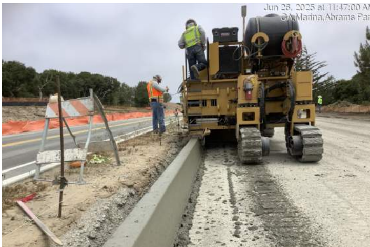
Curb extruding equipment places concrete for median curb along Imjin Parkway east of Abrams Drive
