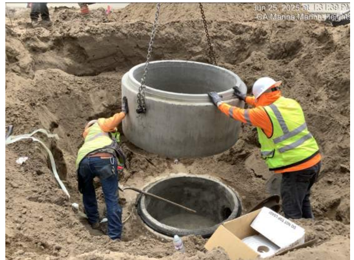
Installing pre-cast manhole sections for drainage facility near Imjin Road
