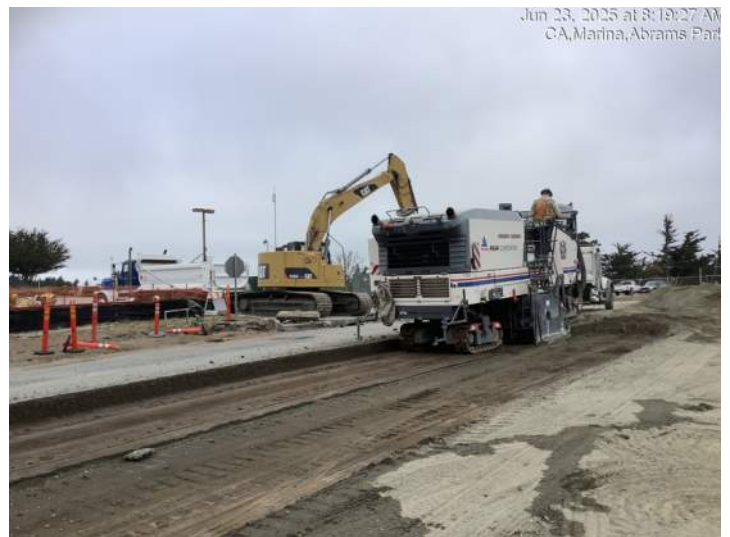
Grinding out remaining pavement on Abrams Drive (south)
