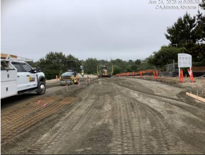
Grading base rock on Abrams Drive (south)
