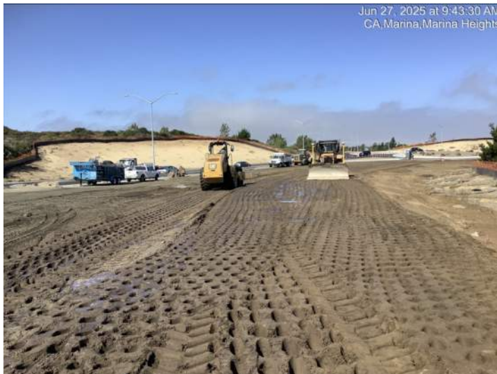
Compacting soil for north roadbed near Imjin Parkway
