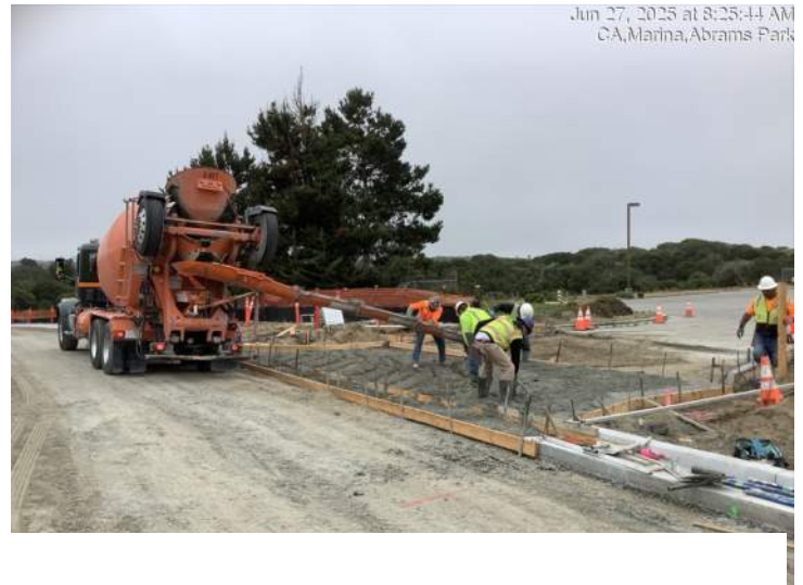
Placing concrete for new driveway at Food & Fuel Mart (Abrams Drive south)
