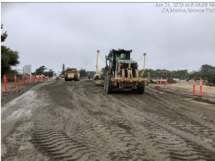
Fine grading operation east of Abrams Drive (south)
