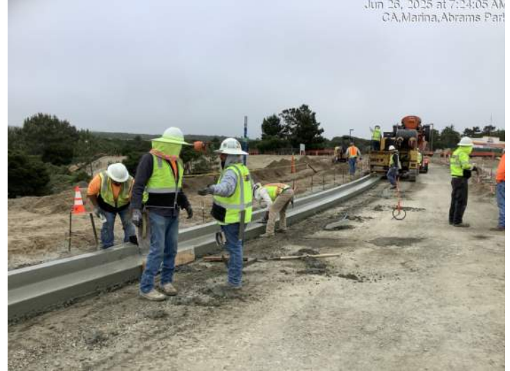
Placing concrete for curb & gutter on Abrams Drive (south)
