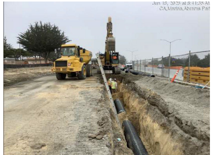
Installing storm drain pipe near Abrams Drive
