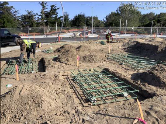
Rebar installed for future art work at Abrams Drive roundabout
