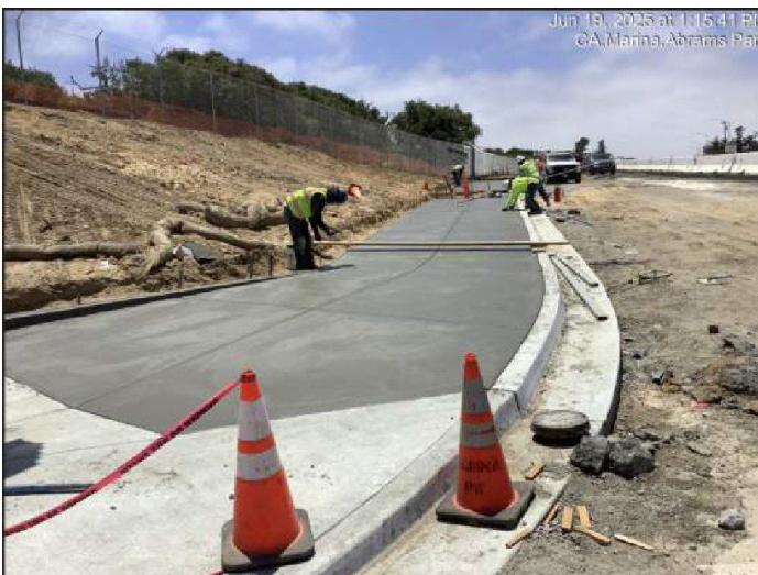
Sidewalk concrete placed near Reservation Road
