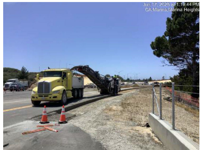
Grinding operation to remove temporary paving near Imjin Road
