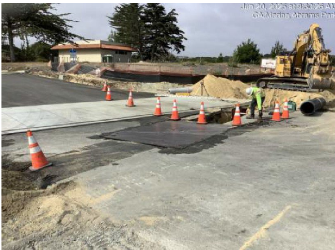
Maintaining business driveway access during pipe installation
