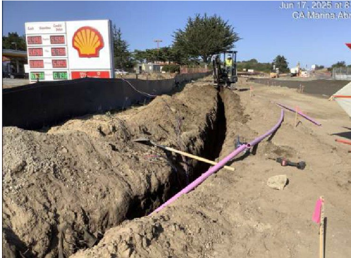
Installing irrigation service lines near Abrams Drive
