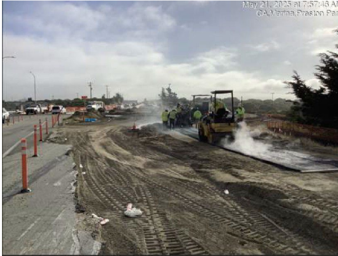
Paving bike path approaching Preston Drive roundabout
