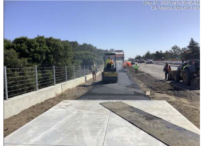
Paving bike path approaching Abrams Drive roundabout
