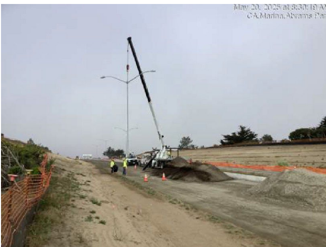
Installing median street light pole
