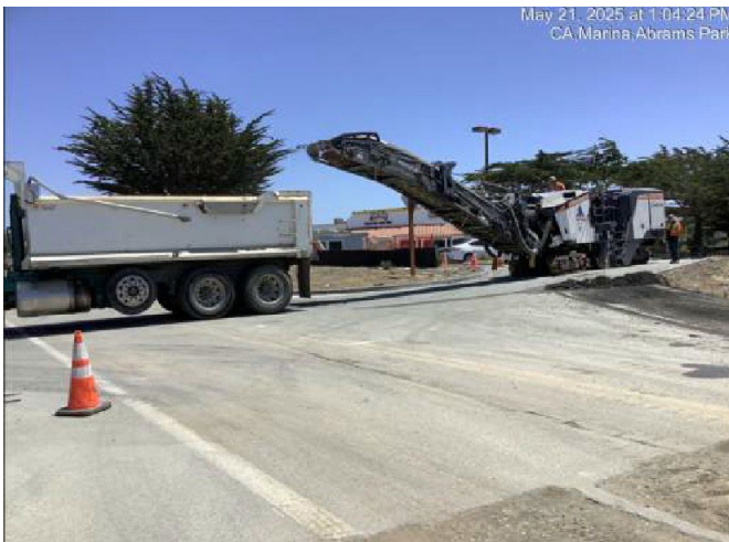
Grinding out existing asphalt driveway at Shell station to make way for new driveway construction
