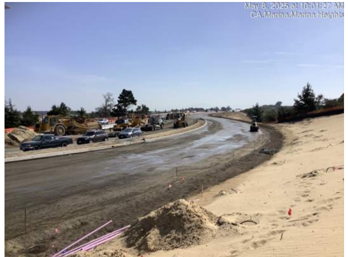
Imjin Parkway (east of Imjin Road) - Fine grading of base rock in preparation for grading
