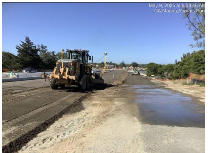
Abrams Drive (north) - Fine grading of base rock in preparation for paving
