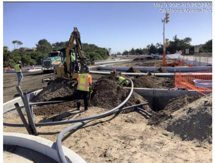
Abrams Drive (north) - Installing electrical conduit for streetlights and flashing beacons (pedestrian crossings)
