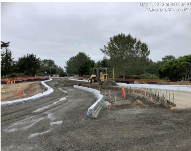
Abrams Drive (north) - Median concrete curb (left) and forming for concrete median curb (right)
