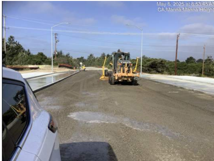
Imjin Road - Fine grading of base rock in preparation for grading
