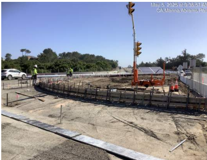
Abrams Drive (north) - Forming for 1/2 roundabout truck apron
