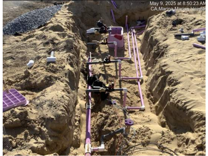
Installing irrigation (for plant establishment) near Imjin Road
