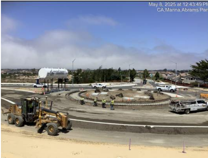
Marina Heights Drive - Forming for 1/2 roundabout (south)
