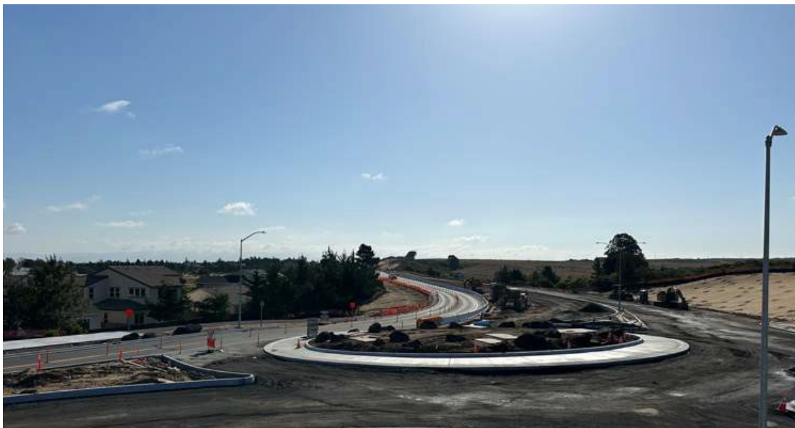
Imjin Road roundabout with completed truck apron and boulders installed
