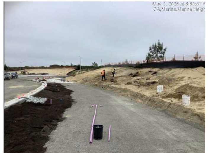
Bioretention soil material in foreground; preparing plant pits on slope in background
