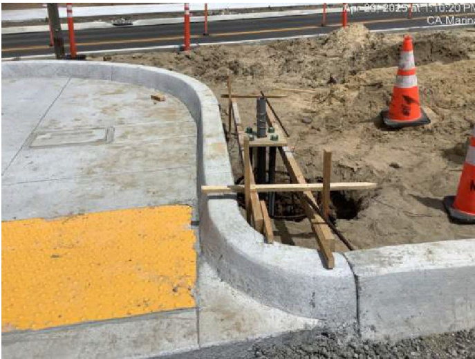
Forming/template for flashing beacon pole bolts/foundation at Imjin Road
