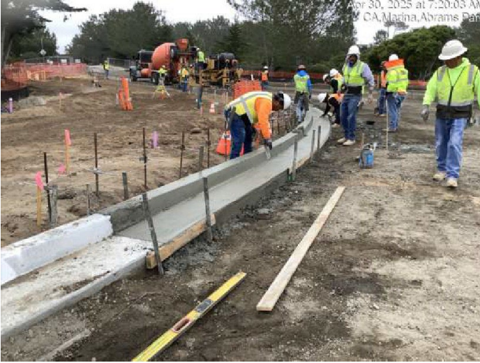
Finishing curb & gutter concrete at Abrams Drive (north)
