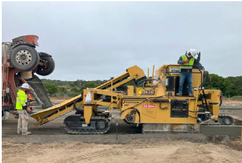
Curb extrusion machine placing curb and gutter at Preston Drive (south)
