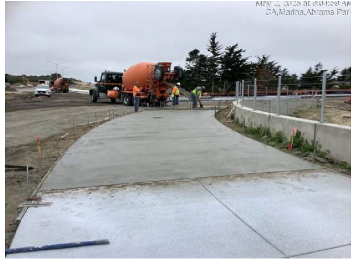
Finishing sidewalk concrete at Abrams Drive (north)
