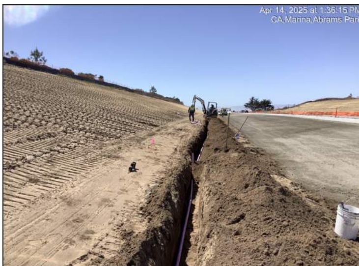
Installing irrigation service lines for irrigation (during plant establishment period)
