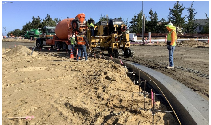
Placing curbing by machine
