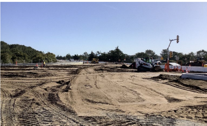
Grading Abrams North side roundabout
