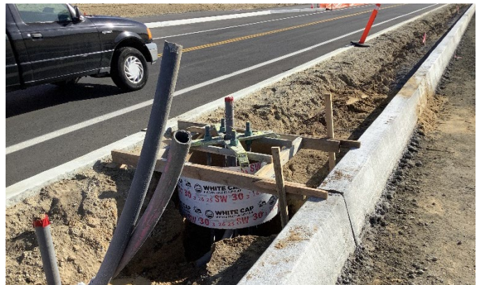
Placing street light foundation
