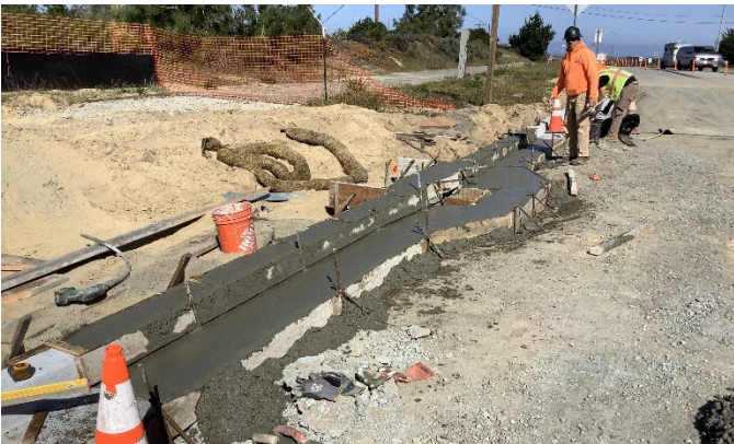
Curbing and storm drain inlet
