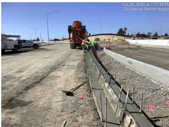
Curb and gutter forms/concrete along Imjin Parkway east of Imjin Road
