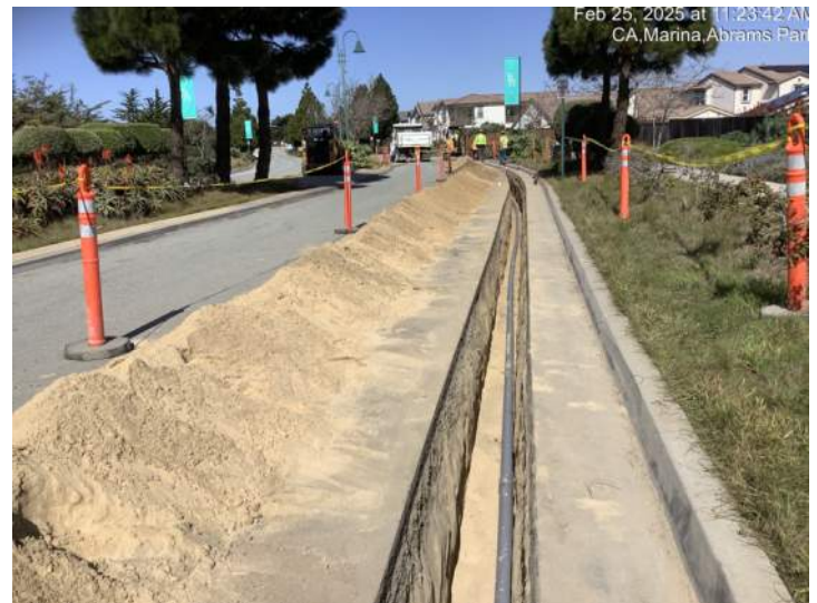
Installing electrical conduit in trench along Marina Heights Drive. This conduit will carry wiring for street lights and irrigation controller service.
