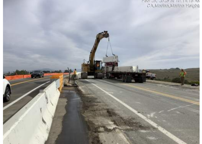
Loading out concrete barrier rail used in Phase 1
