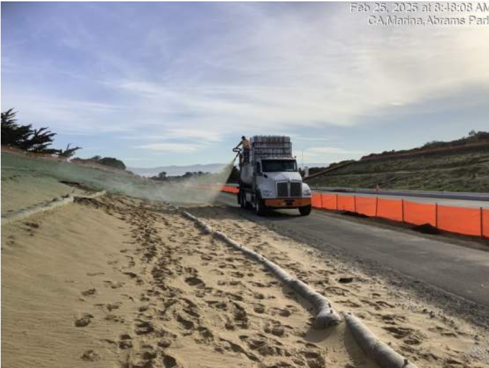
Hydroseeding slopes along Imjin Parkway for erosion control
