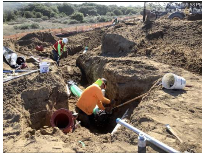
Last segment of pipe for relocated sanitary sewer force main (across from Preston Drive)
