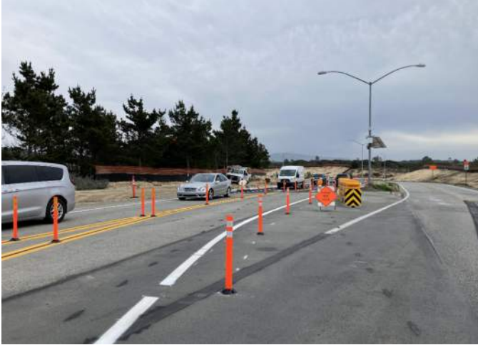
Traffic shift onto new pavement on north roadbed for Phase 2 construction
