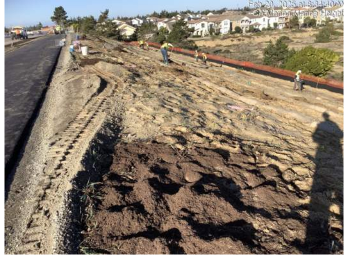
"Prepping" plant pits - digging holes and placing gopher protection cages and specified soil mix for future plantings
