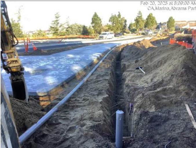
Installing electrical conduit along Marina Heights Drive
