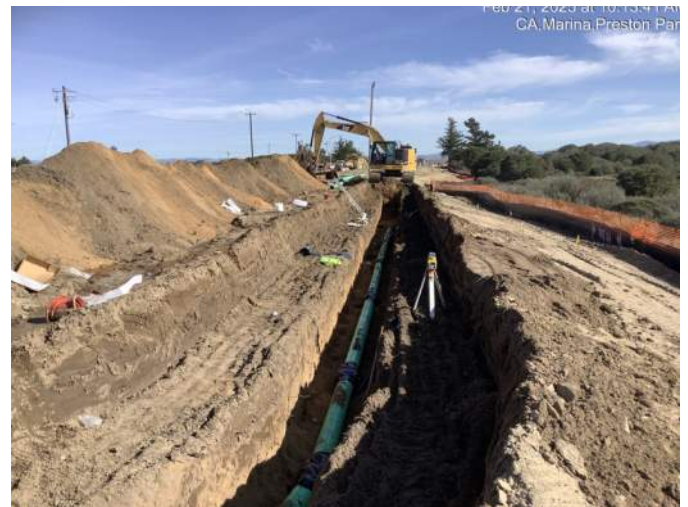
Installing new pipe to re-route conflicting MCWD sewer force main (across from Preston Drive)
