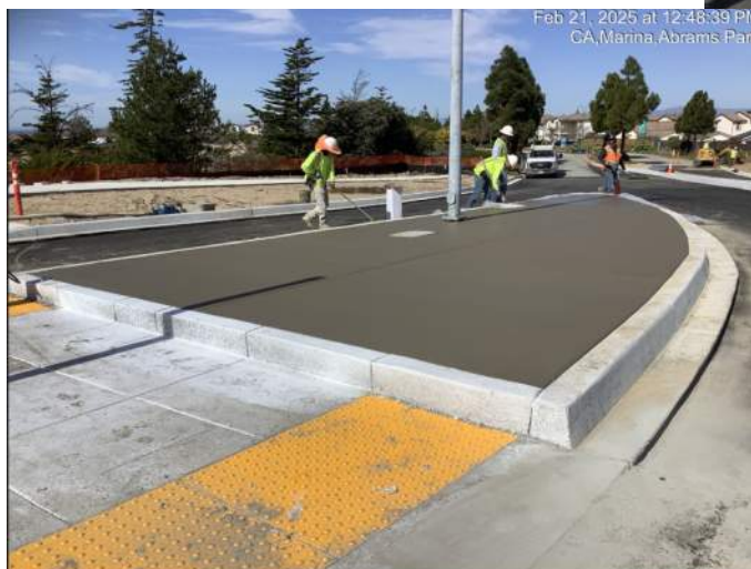
Finishing concrete median at the top of Marina Heights Drive
