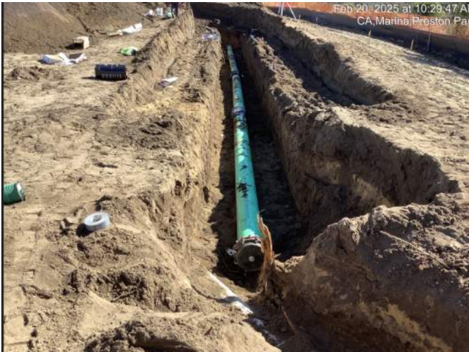
Installing new pipe to re-route conflicting MCWD sewer force main (across from Preston Drive)
