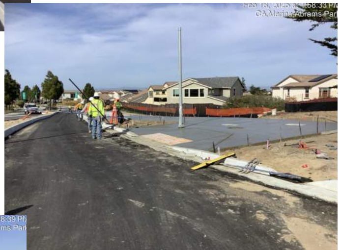
Finishing concrete sidewalk(s) along Marina Heights Drive
