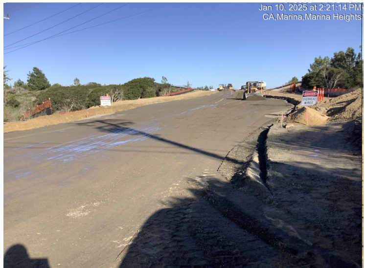
Earthwork/grading operations on Imjin Road
