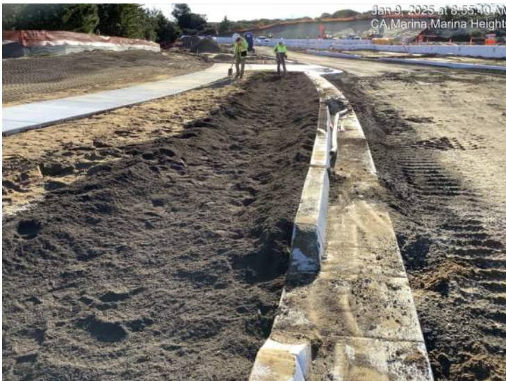
Special soil material installed for bioswales
