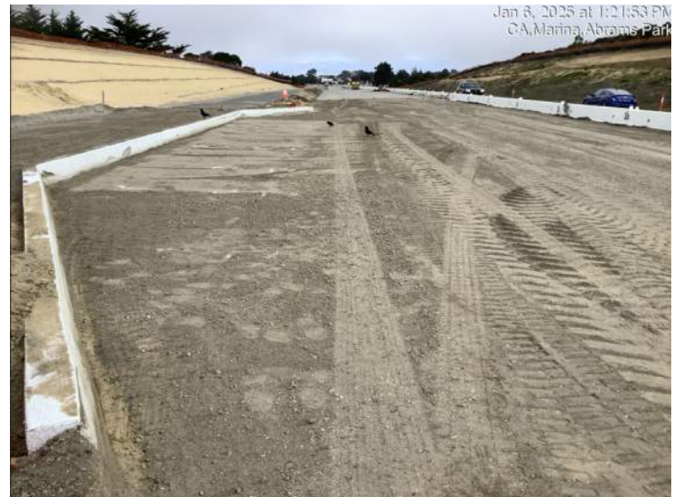
Finished grade (ready for paving) east of Marina Height Drive
