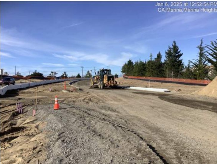
Fine grading operation west of Marina Height Drive
