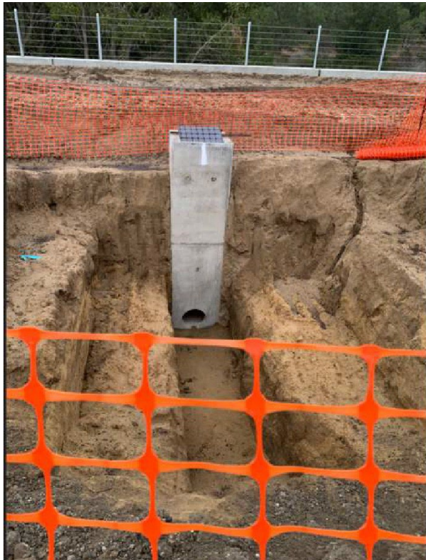
DAY WORK & NIGHT WORK INSTALLING STORM DRAIN CROSSING UNDER IMJIN PARKWAY AT THE RETAINING WALL NEAR ABRAMS DRIVE
