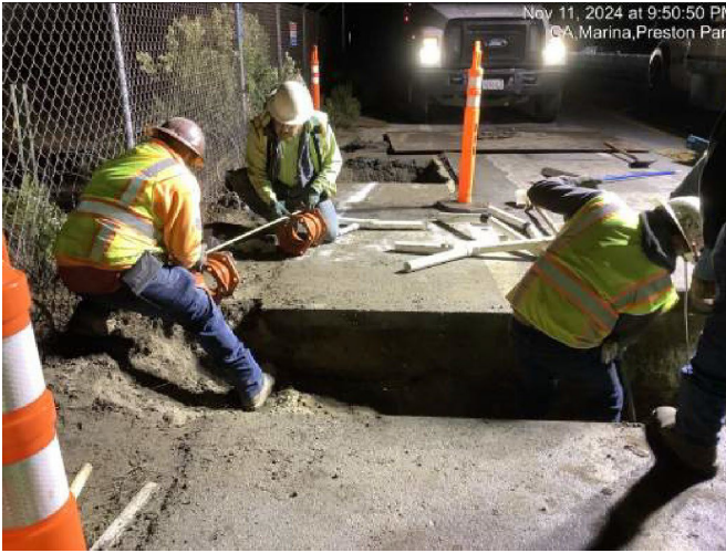
NIGHT WORK INSTALLING WATER SERVICE CROSSING IMJIN PARKWAY FOR ARMY RESERVE & CHAPIN YARD
