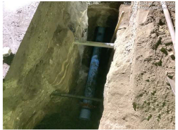
NIGHT WORK INSTALLING WATER SERVICE CROSSING IMJIN PARKWAY FOR ARMY RESERVE & CHAPIN YARD
