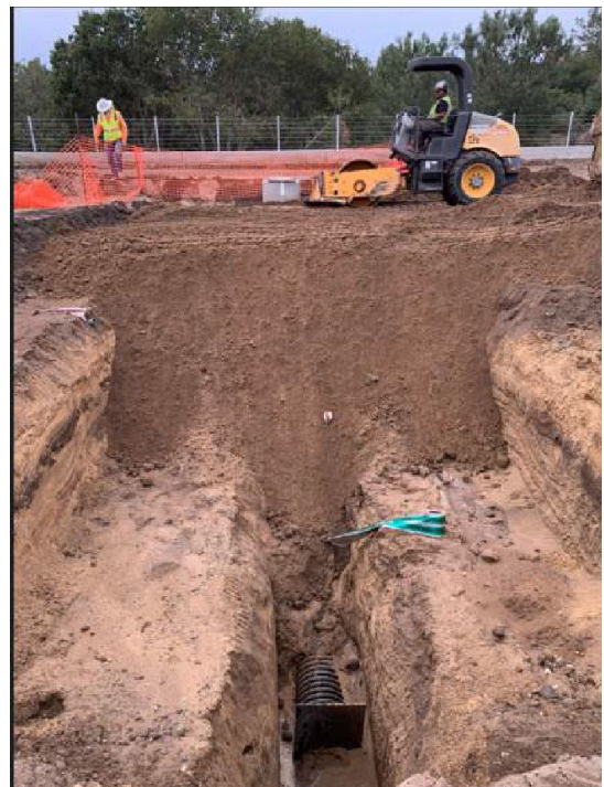
DAY WORK INSTALLING STORM DRAIN CROSSING IMJIN PARKWAY NEAR ABRAMS DRIVE
