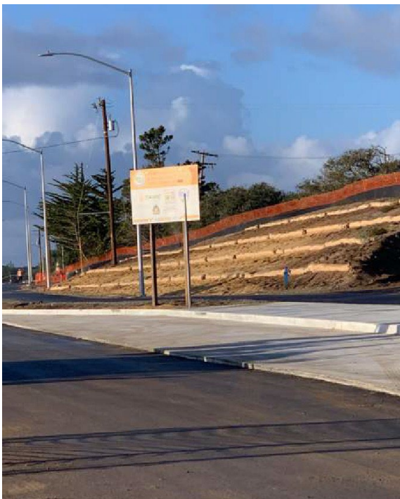
STRAW WADDLES INSTALLED ON SLOPES TO PREVENT EROSION IN RAIN EVENTS
