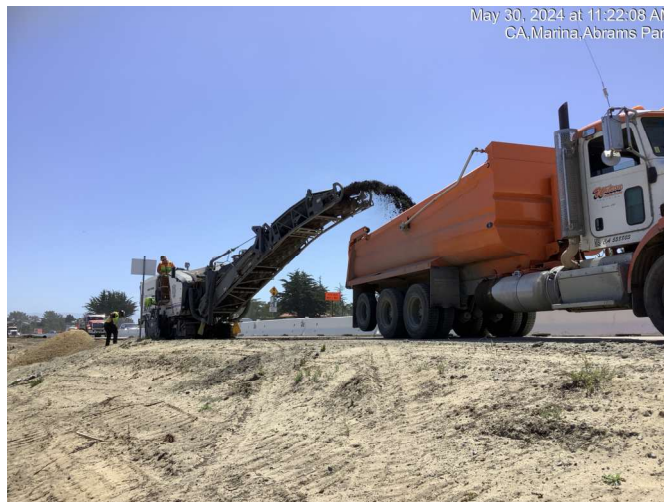
Grinding out/removing existing pavement near Marina Heights Drive
