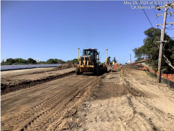
Grading equipment levels out earthwork fill near Reservation Road
