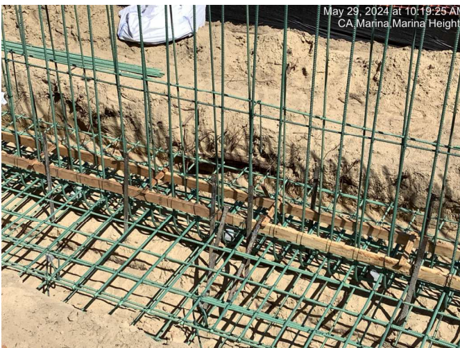
Bar reinforcing steel installed for retaining wall footing and wall near Marina Heights Drive
