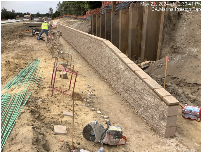
Completing work on small retaining wall near Preston Drive
