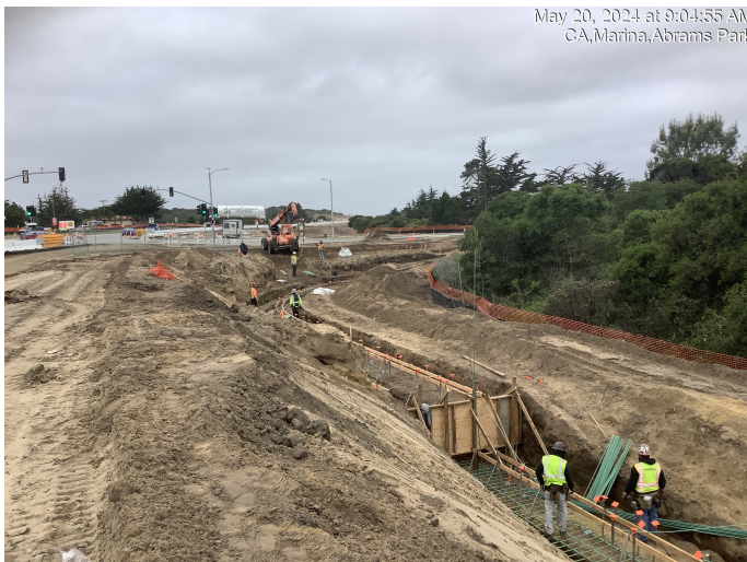
Installing bar reinforcing steel and forming for retaining wall near Abrams Drive
