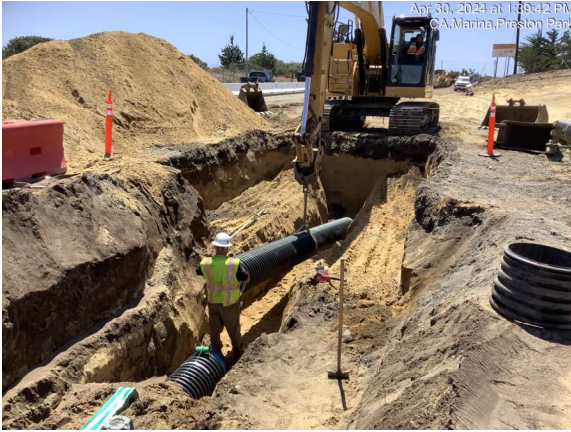
Storm drain installation near Reservation Road
