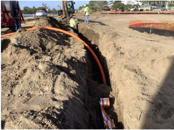
Installing fiber optic conduit near Preston Drive
