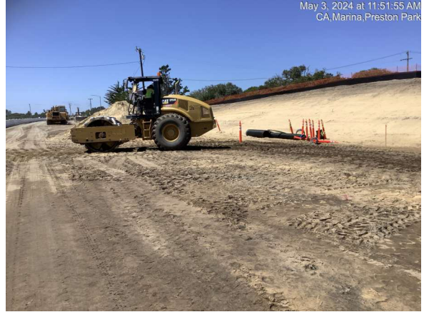
Compacting earthwork fill near Reservation Road
