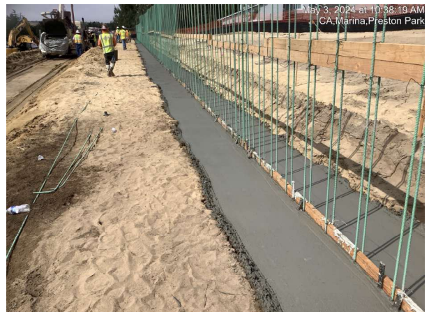
Concrete for retaining wall footing adjacent to Preston Park
