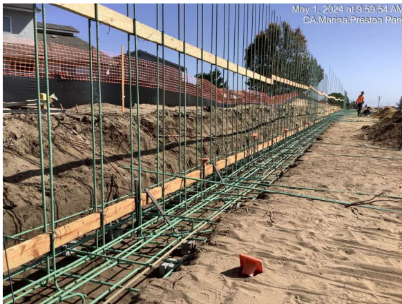
Reinforcing steel for retaining wall adjacent to Preston Park
