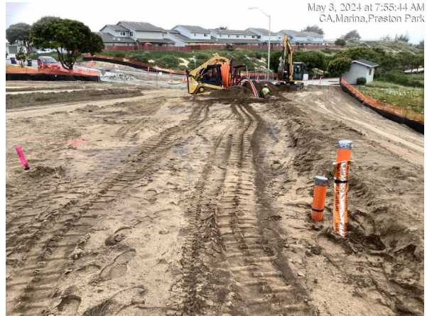
Fiber optic trench backfilled and compacted
