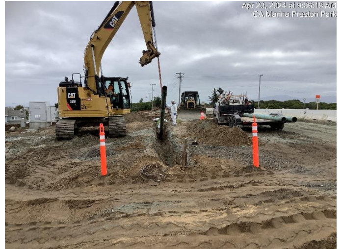
Removal of abandoned utility pipe near Preston Drive
