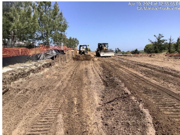
Continued Roadway grading and earthwork Between Preston and Abrams
