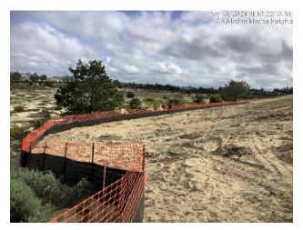
Continued installation of silt fencing on project perimeters
