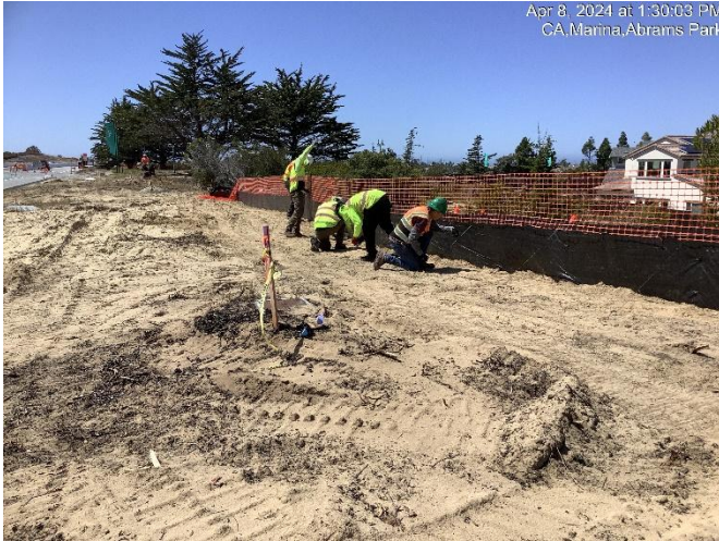
Continued installation of silt fencing on project perimeters
