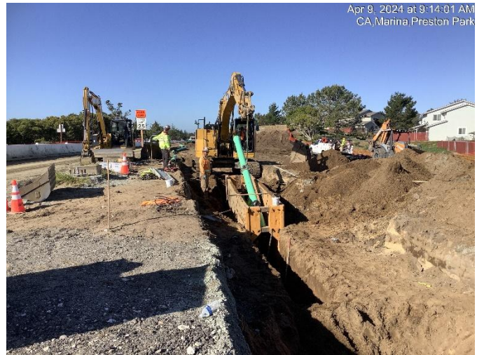
Continuing installation of new sanitary sewer line at Preston Drive
