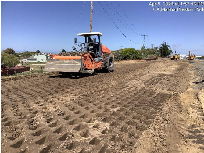
Roadway grading and earthwork by Preston Drive
