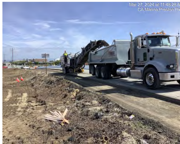
Grinding and removal of old roadway pavement
