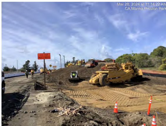
Earthwork operations near Reservation Road - cutting and filling dirt to achieve grades for new roadway
