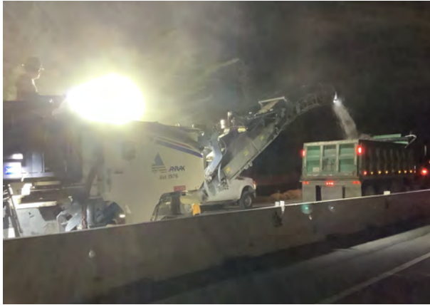
Night work - grinding pavement in pothole locations
