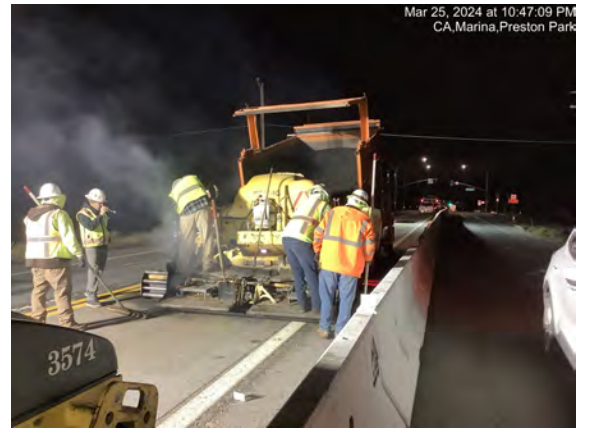
Night work - new pavement in pothole locations
