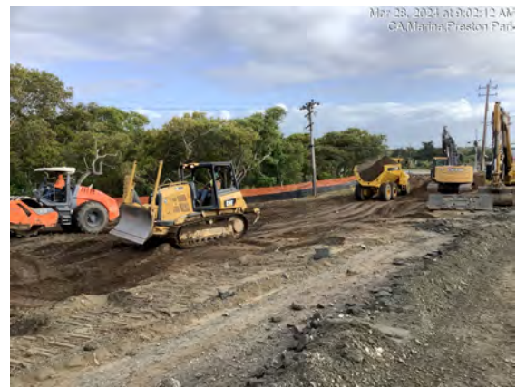
Earthwork operations near Reservation Road - cutting and filling dirt to achieve grades for new roadway
