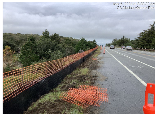
Silt/High-Visibility Fencing Installation
