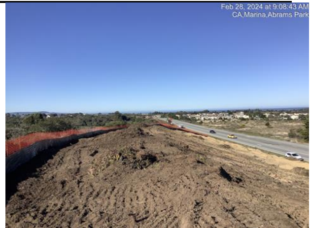
Looking west - tree & brush removal along eastbound side
