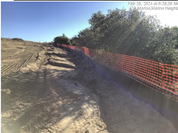
Installing perimeter silt fence
